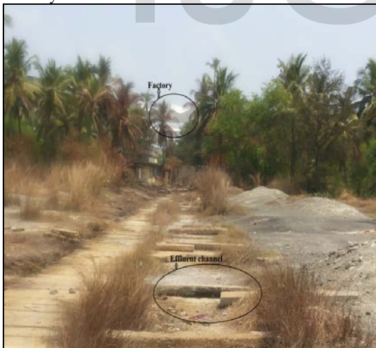
Fig3. Effluent Channel from factory
